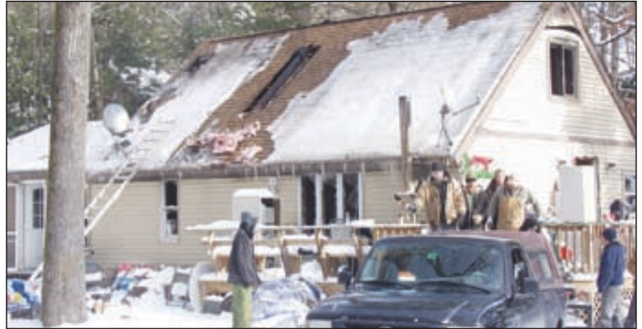
This house on Spring Street was a total loss.
