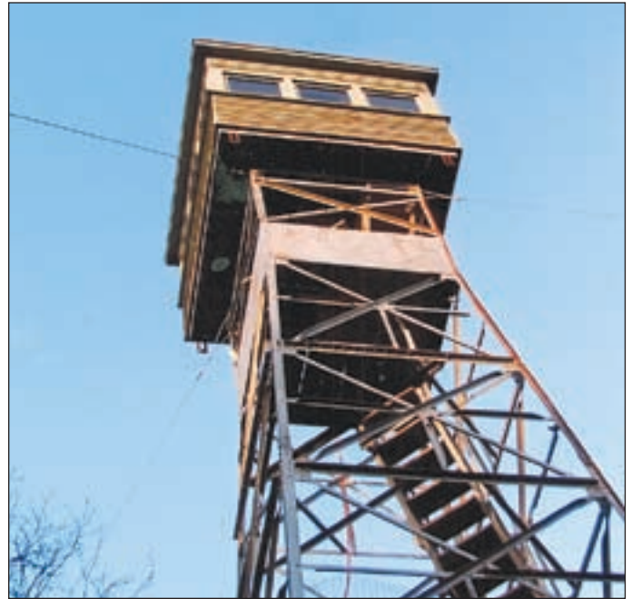
The Craney Hill Fire Tower.
