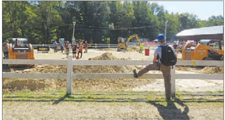
NH Construction Career Days was held on the 4-H Fairgrounds in New Boston.
