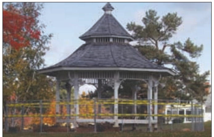
Repairs are underway at New London's Mary Haddad Bandstand.
