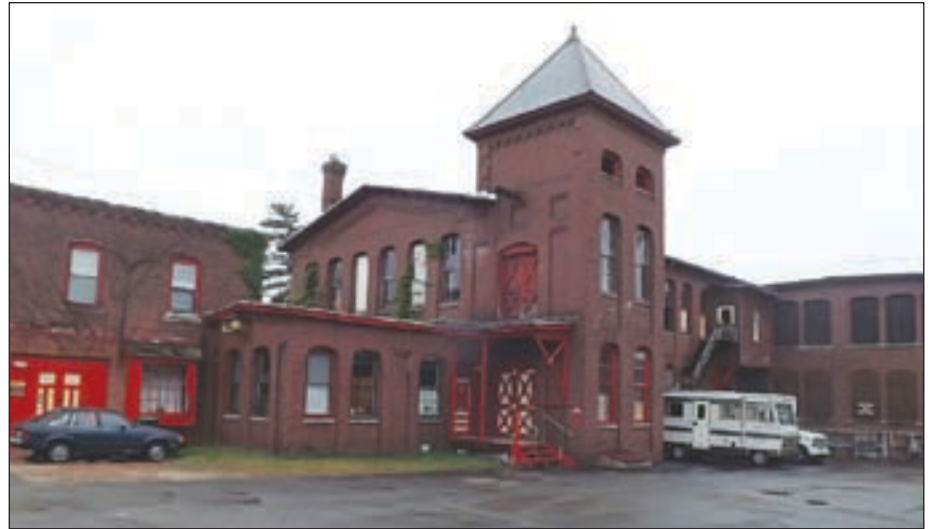
Major improvements are planned for this Franklin Mill.
