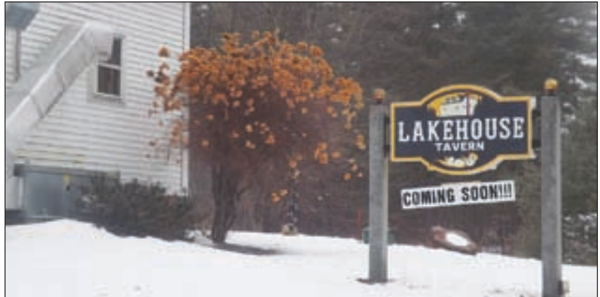
With extensive renovations nearing completion, Hopkinton's newest restaurant, The Lakehouse Tavern should be opening soon.
