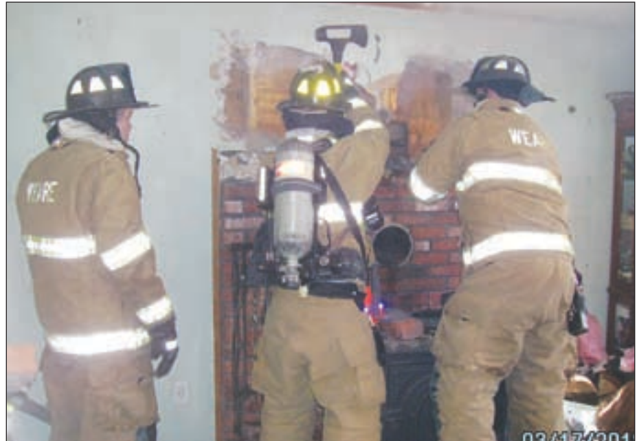
Weare firefighters break through the wall to get to the fire.
