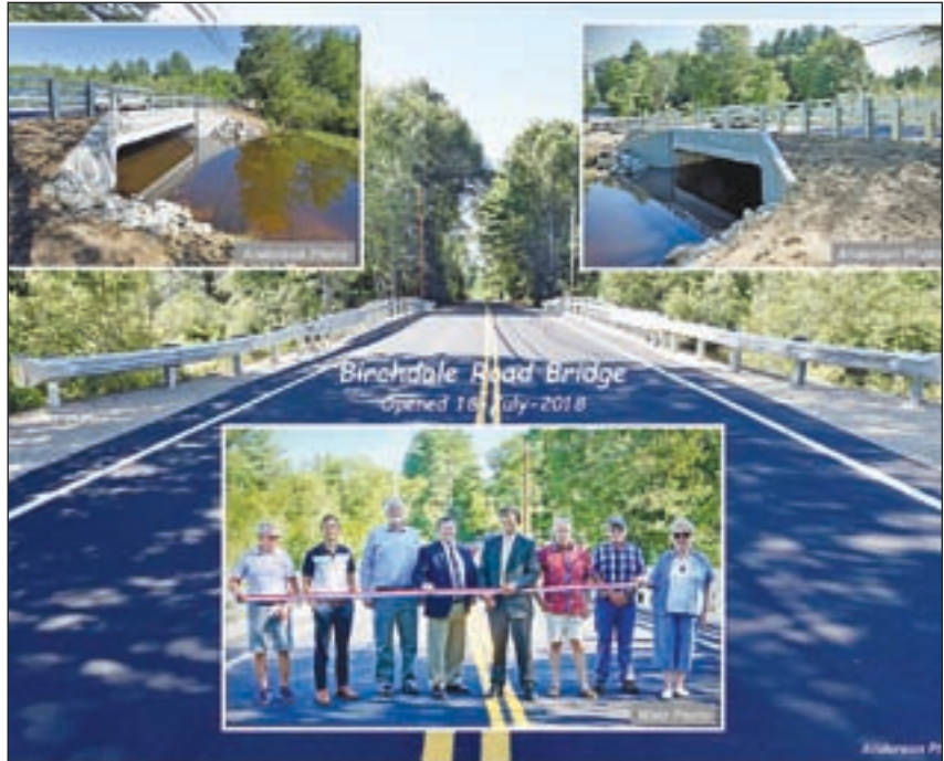
Closed for three years, Bow's Birchdale Road bridge rebuilt & reopened.
