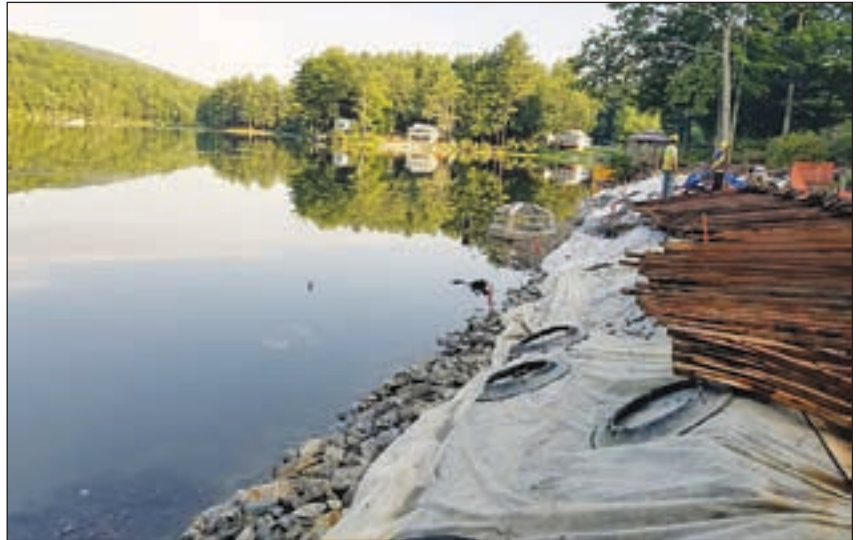
Work is progressing on the Uncanoonuc Dam Project.
