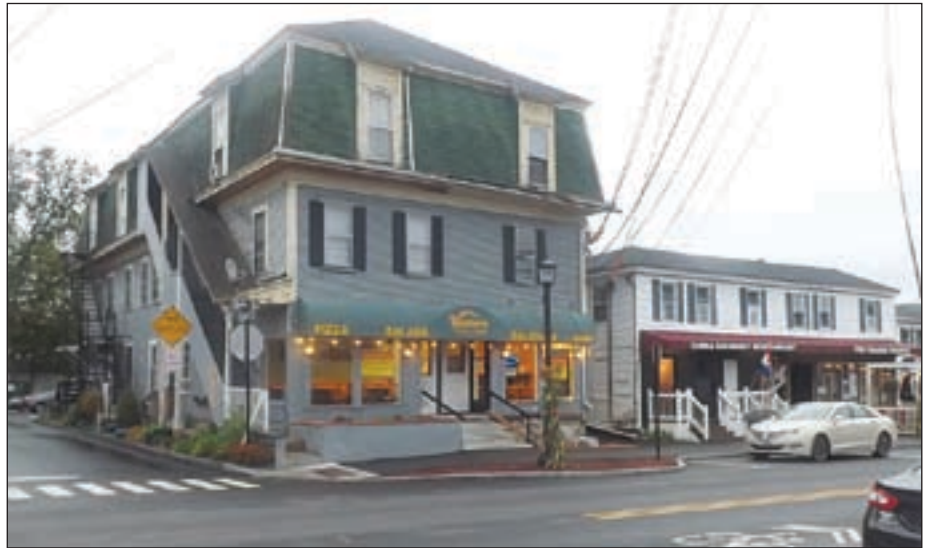
Tax incentives will contribute to a renovation of this building.
