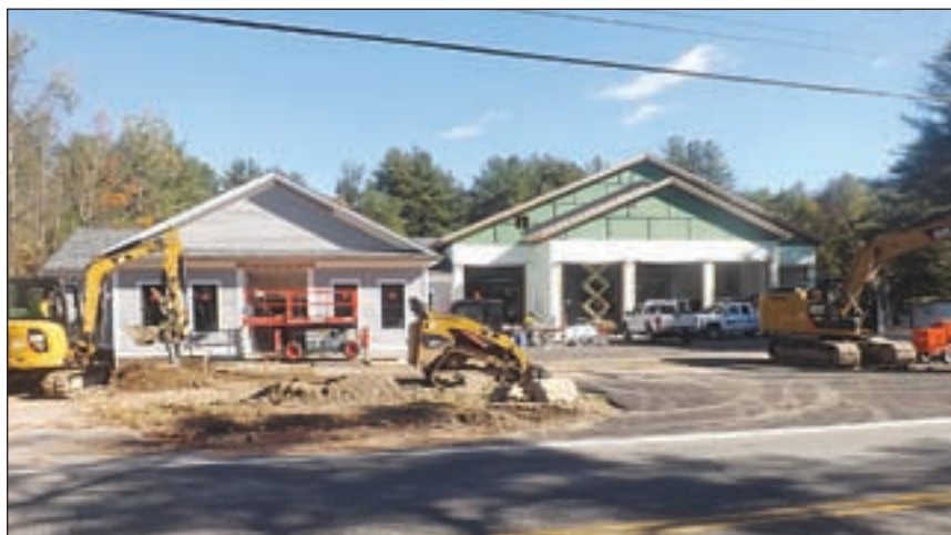
Work is proceeding in Warner's new Fire Station.
