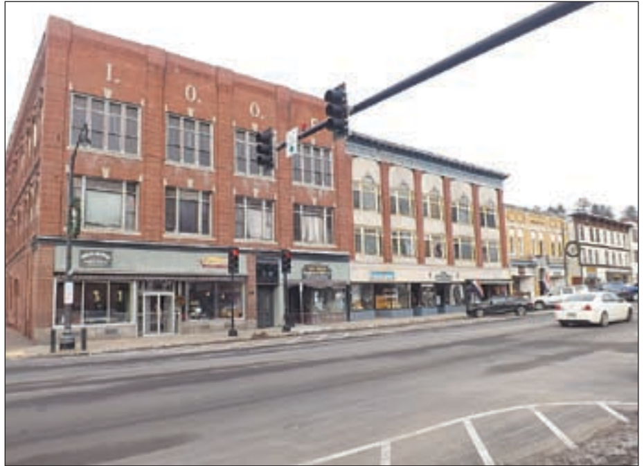
These Central Street buildings will soon receive a major renovation.
