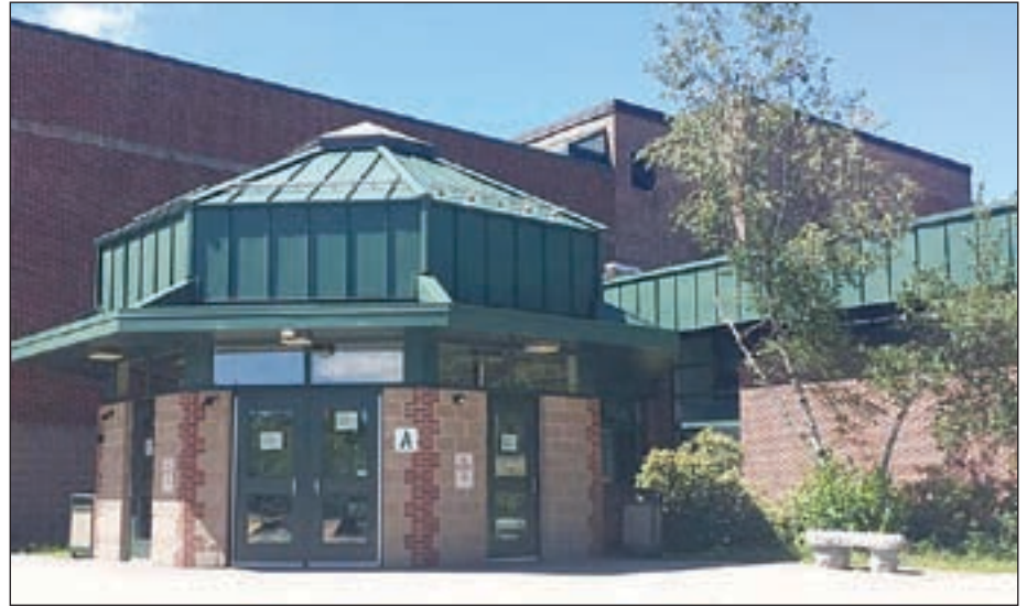
School Board reports that Hopkinton schools have many deferred maintenance issues.
