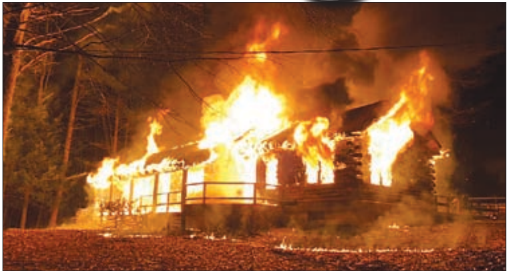
Peterborough Firefighters battled a fire at a vacant home being renovated on Carley Road early Monday. The fire started sometime before 5 a.m. and was knocked down just after 6 a.m. No injuries have been reported.
