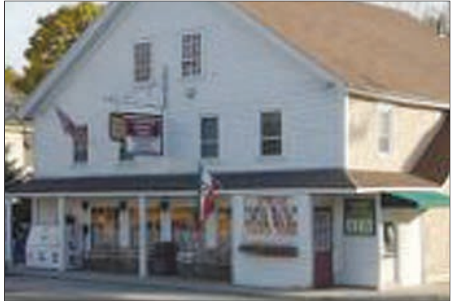
The Cracker Barrel store will soon be renovated.
