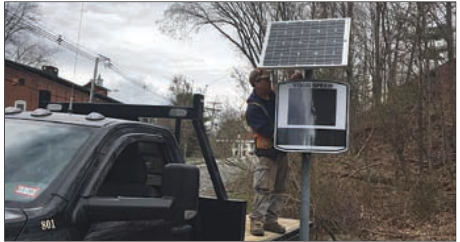
Antrim has just installed a digital speed sign on Main Street coming into town from Bennington. You will notice a digital read out of your speed when approaching the sign. Green numbers indicate a second digital speed sign near Mush Cooks Garage will be installed in the future.
