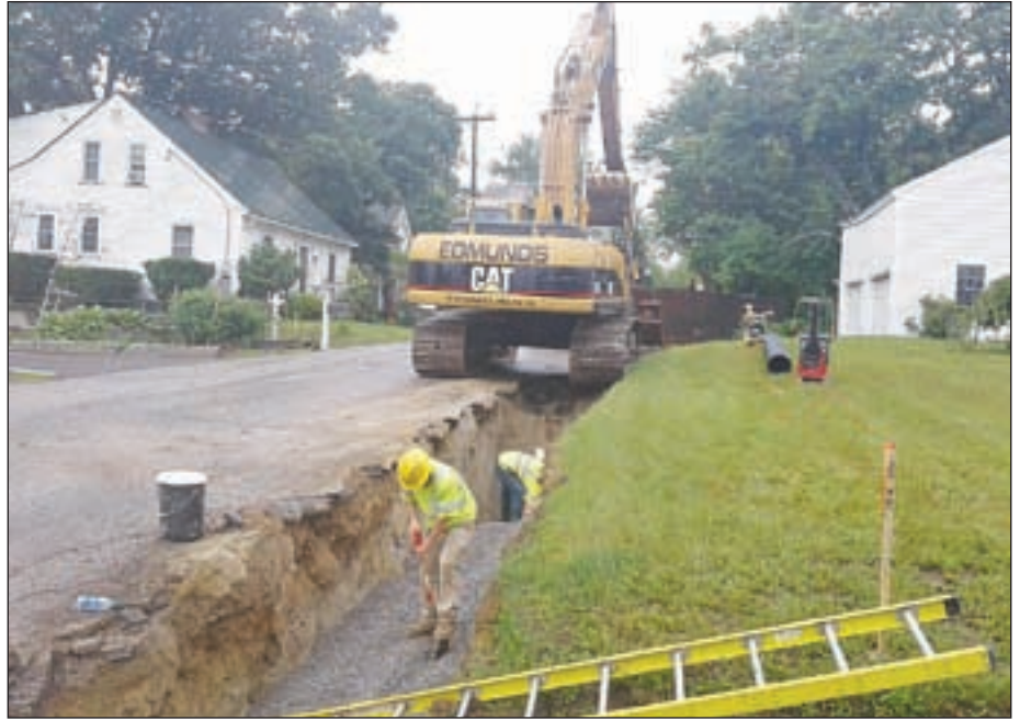
Crews have begun replacing the water mains on Hall Avenue.
