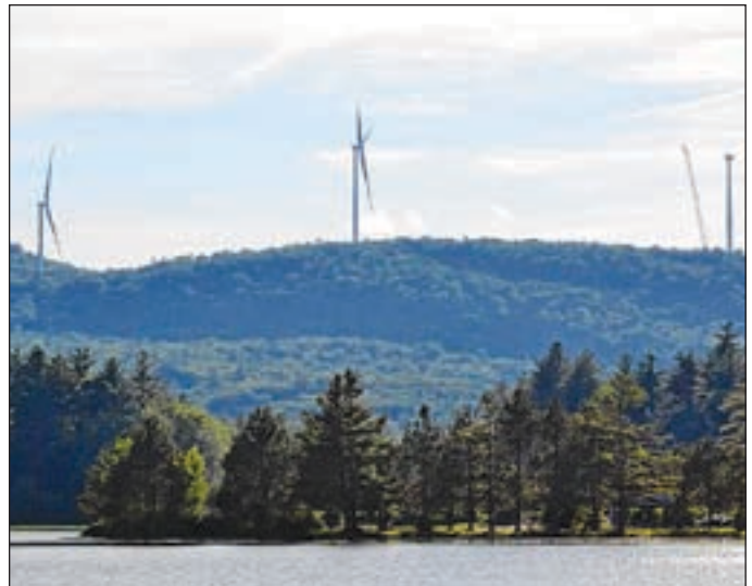
A view of the new wind towers from Gregg Lake Beach. Courtesy photo.
