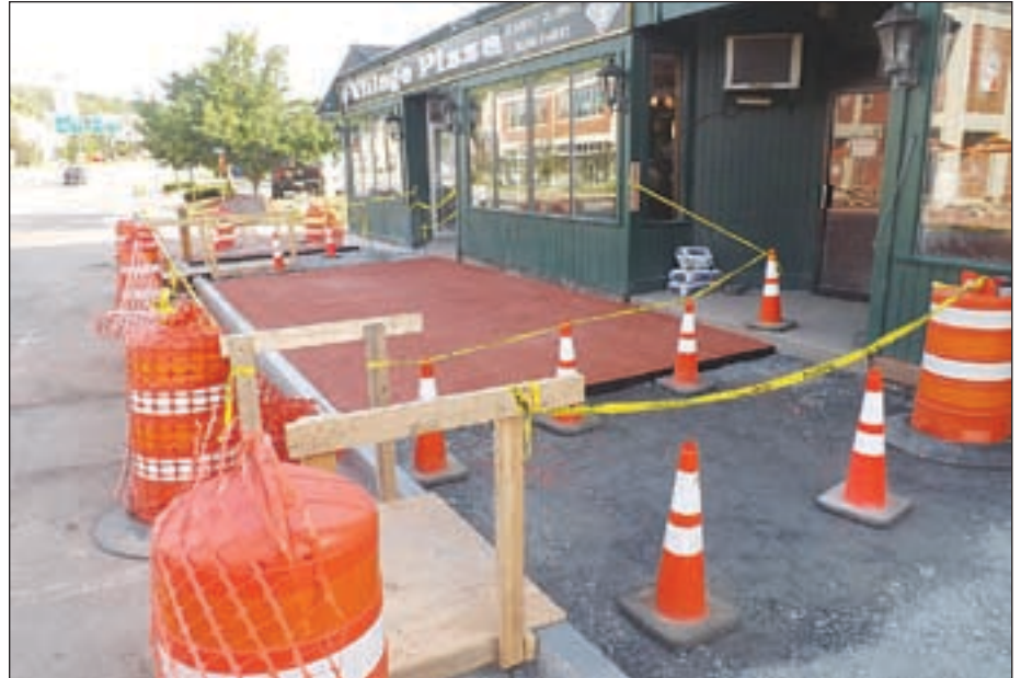
A major sidewalk renovation project is underway in Newport.
