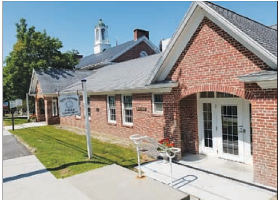
North Branch Construction Completes New London Police Station Renovations.
