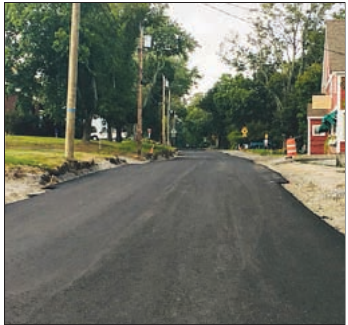
Hennikers ambitious highway, sidewalk and drainage projects are continuing on schedule.
