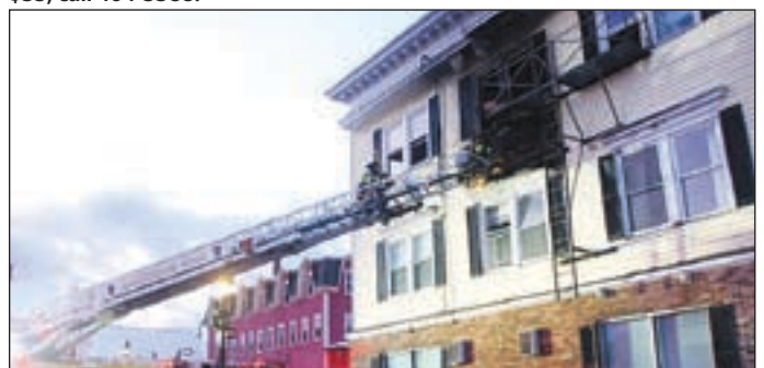
Quick action by Henniker Fire and Rescue extinguished the fire. A special thanks to Abby Myskowski, the owner of St. George's Cafe. Abby called 911 and alerted the occupants of the building.
