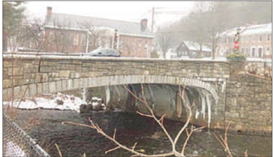
Repairing this bridge will cost $1.6 million more than expected
