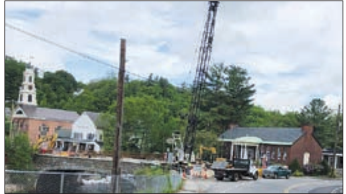
Work is progressing on replacement of Peterborough's Main Street bridge.
