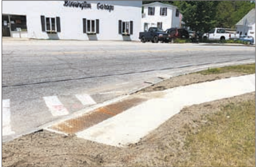
Downtown Bennington had ADA-compliant ramps and bump strips installed on its sidewalks last week. The update was a stipulation of NH DOT's road repaving project. Resurfacing of streets constitutes an alteration under the Americans with Disabilities Act (ADA), so it requires curb ramps where pedestrian walkways intersect the resurfaced streets.
