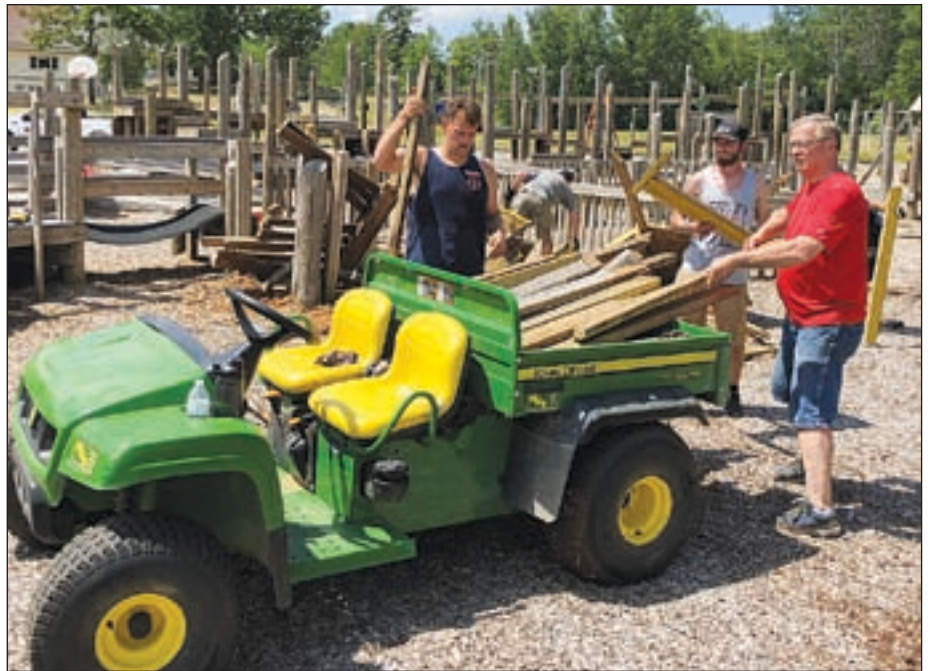
Workmen with power tools have begun the demolition.
