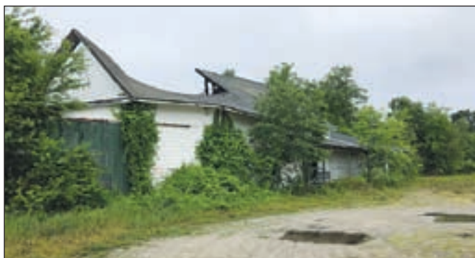
Non-use and neglect have caused the demise of Hillsborough's original Railroad Station.
