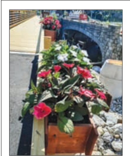
Thanks to a small but dedicated group of green-thumbed Peterborough volunteers, two flower boxes have been installed on the temporary pedestrian bridge.
