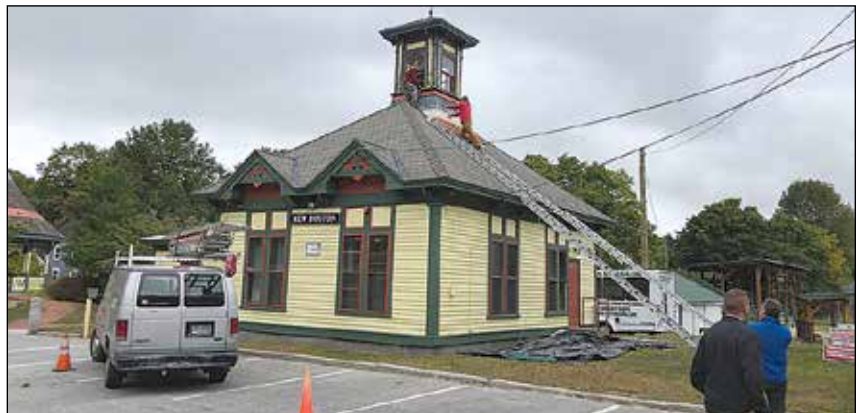
Cupola repairs are being completed in New Boston.
