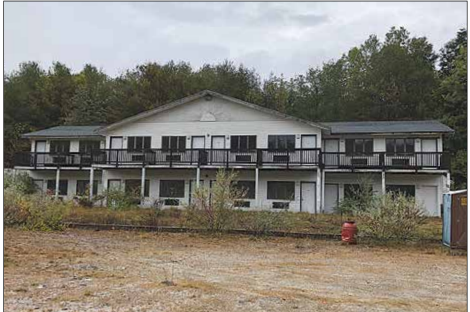
The former Highland Inn is receiving a second life.
