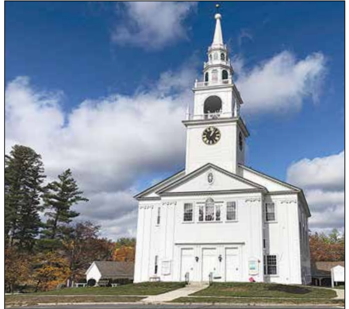
The historic Hancock Meetinghouse has survived for just over two centuries since its dedication on October 25, 1820. It remains as only one of NH meeting houses that is utilized by both the town and a church. The building is actually the town's second Meetinghouse, as the original, built in 1789, was destroyed by fire. The Corona-19 pandemic has delayed any plans for a celebration.
