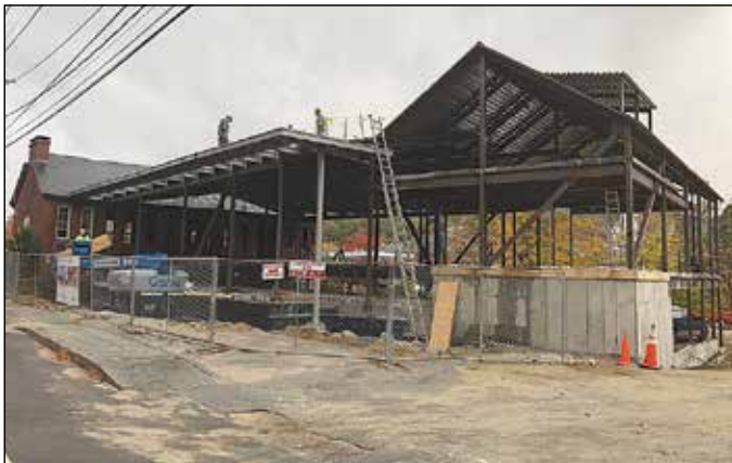
The major addition to the Peterborough Library is progressing on schedule.
