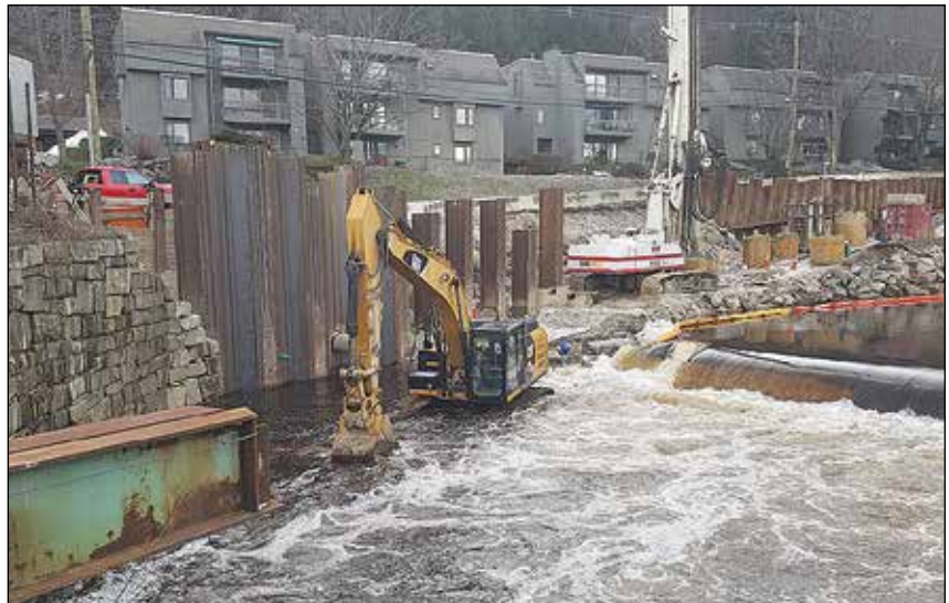
Peterborough construction crews had to wait for the river to subside before pumping down the water in the west cofferdam to gain access and resume working. The flooding will not delay the overall schedule of the Main Street Bridge project.
