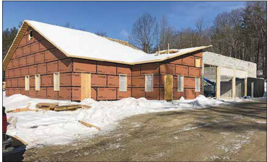
Progress continues on Newbury's new Fire Station.
