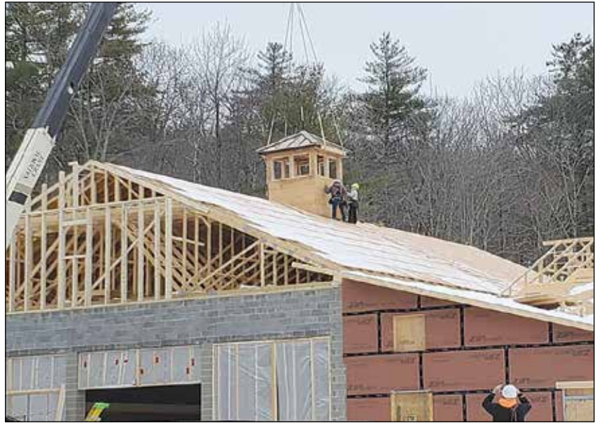
The cupola has been installed on Newbury's new Fire Station.
