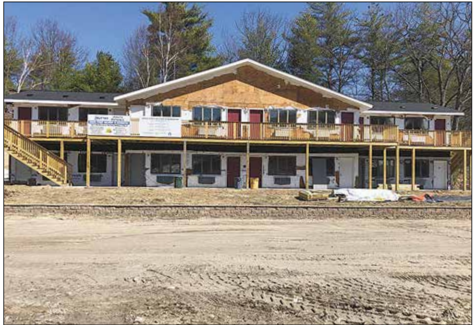
The former Highland Inn is being converted into a detox center.
