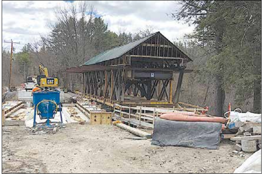
Bridge work has resumed in Bradford.
