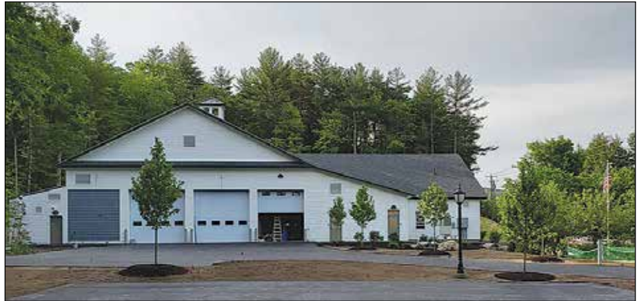
With the project on schedule, officials hope for a dedication in August.
