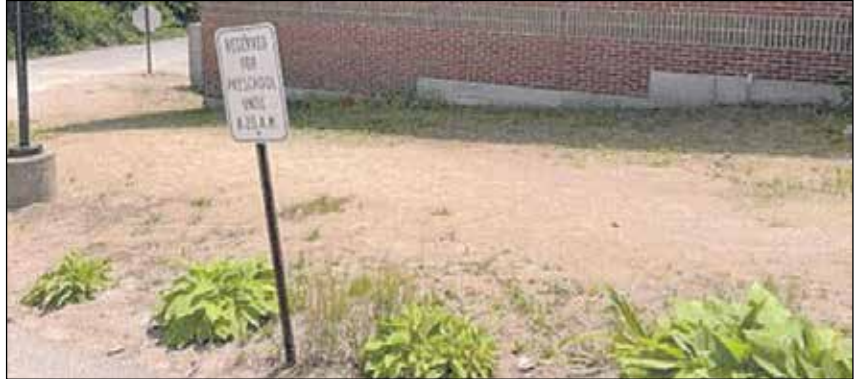
The Hopkinton Public Schools Foundation’s grant was given to turn this space into an outdoor learning classroom at Harold Martin School. Plans include a small retaining wall, fencing around the entire space, a deck, a concrete walkway, and a garden area.
