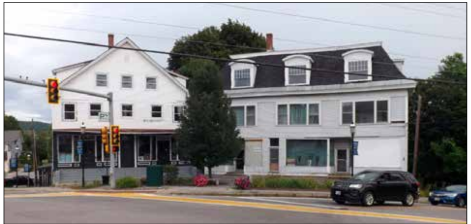
A developer is exploring renovating or replacing these empty buildings.
