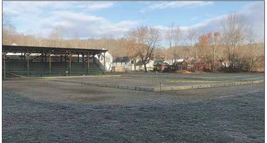
A skating rink is being installed behind Town Hall.
