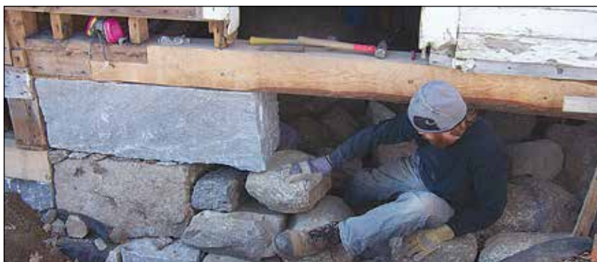
Repairs continue on the Antrim Grange.
