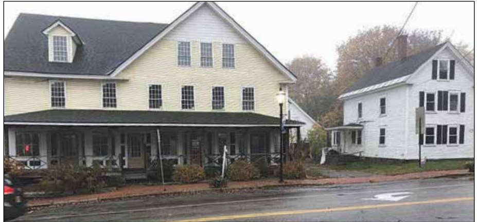
If the ZBA approves, the white building would be torn down and the yellow building converted to apartments.
