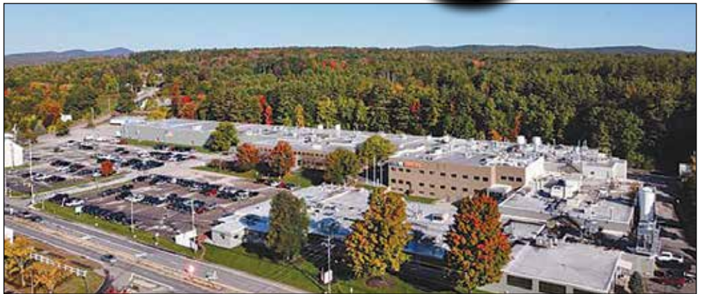
Built for but never occupied as a shoe factory, Sylvania purchased the original building in 1956.
