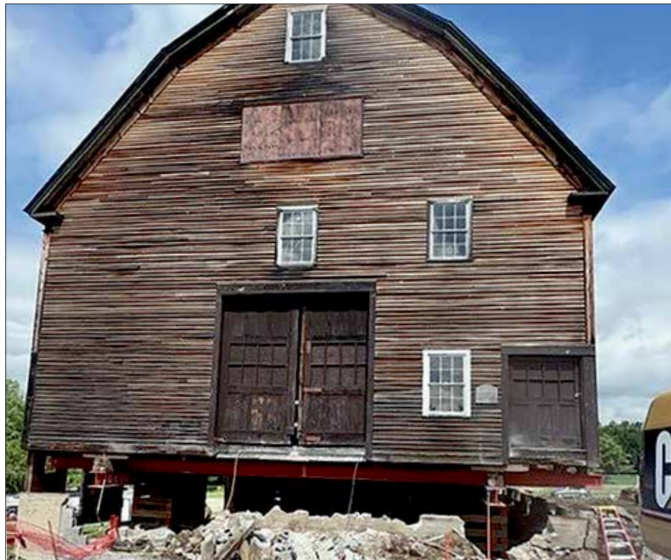
WORKS IN PROGRESS: Renovation of Newbury shared Fire & Police building into the town's new Police station is well under way (left photo). Hopkinton's historic 44' x 100' Houston Barn was raised up about 4 feet off its foundation (right photo). The demolition of the old foundation wrapped up last week. Once the barn has been securely raised, a new foundation will be put in and the barn lowered back into place. It is an impressive undertaking.
