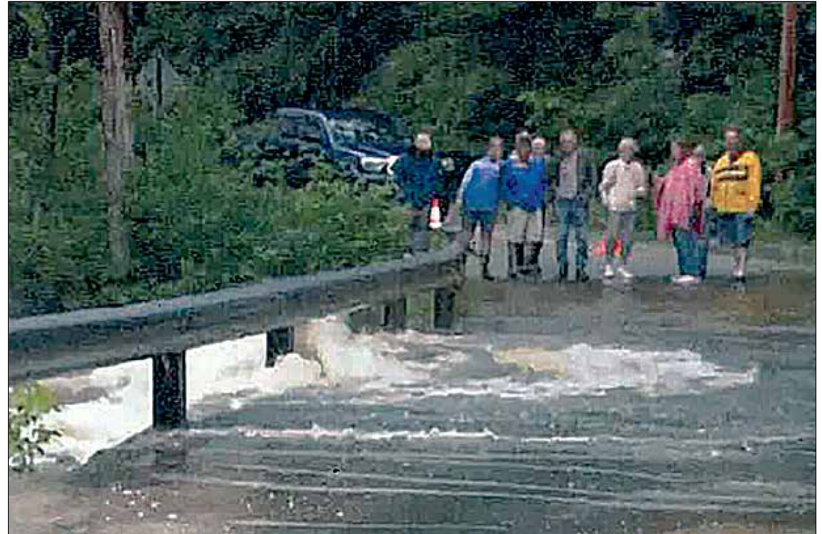
Water pours over Liberty Hill Road in Antrim.
