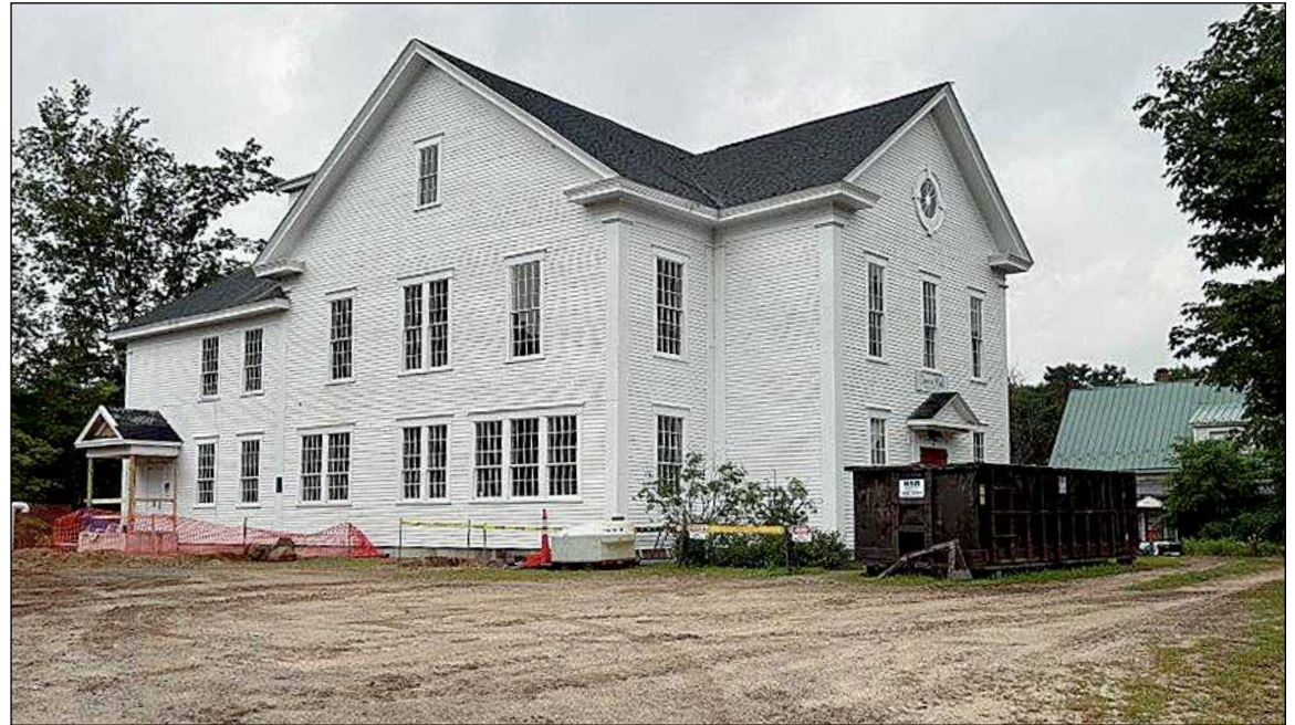
Renovations are nearly complete at Bradford's historic town hall.
