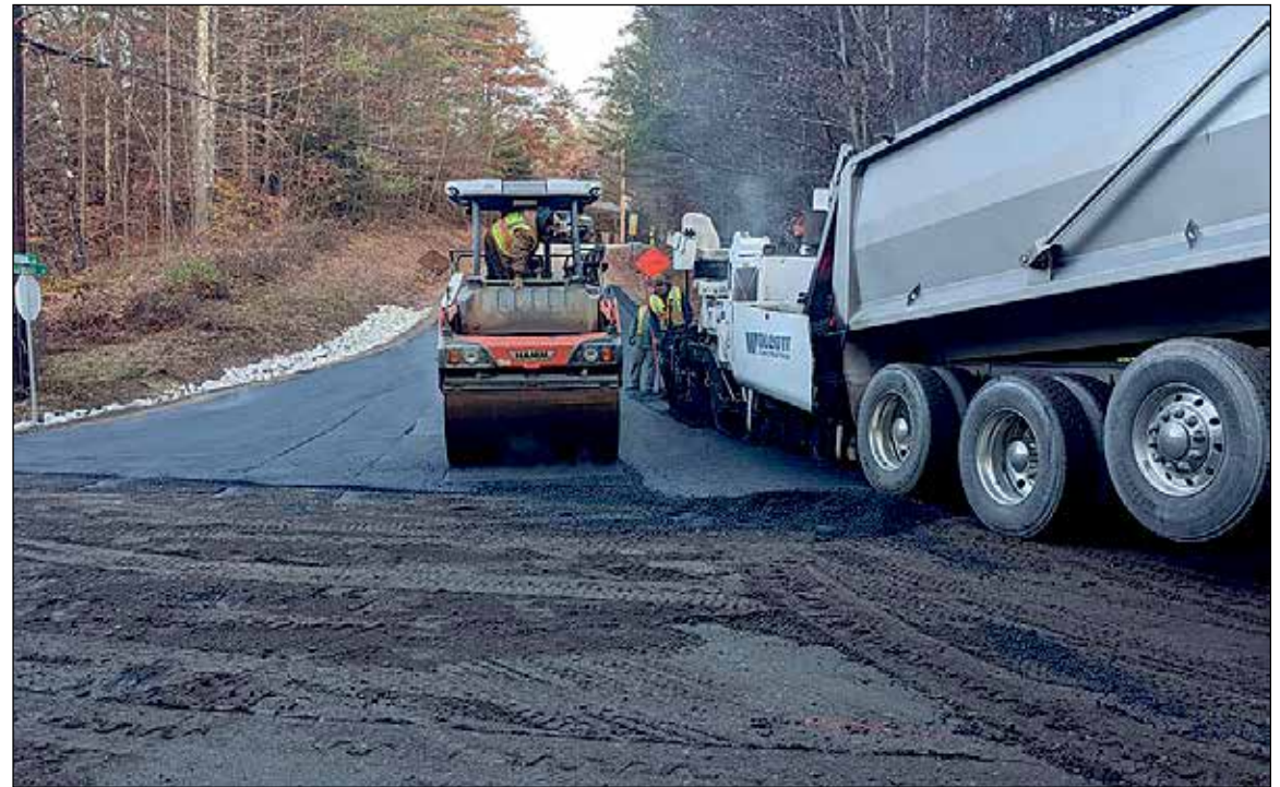
The Henniker Highway Department has started paving Foster Hill! The base coat has been completed. We will return to complete the road and apply a top coat in the spring once things dry out.
