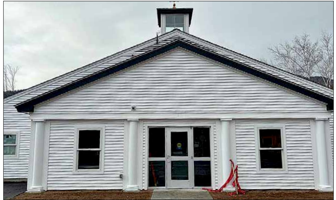
Renovation of Newbury's new Police Facility is nearing completion.
