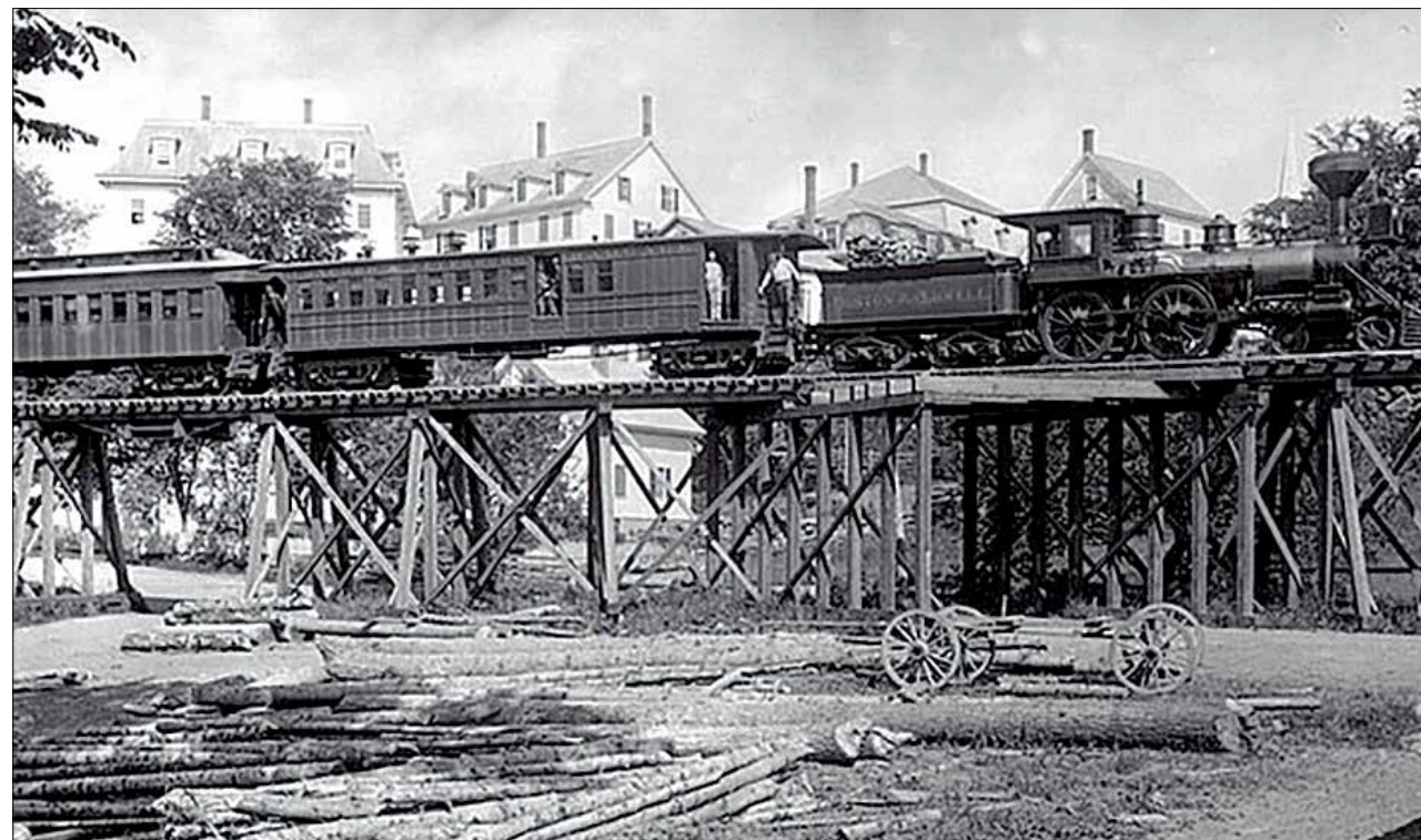
Hillsborough Railroad Trestle
