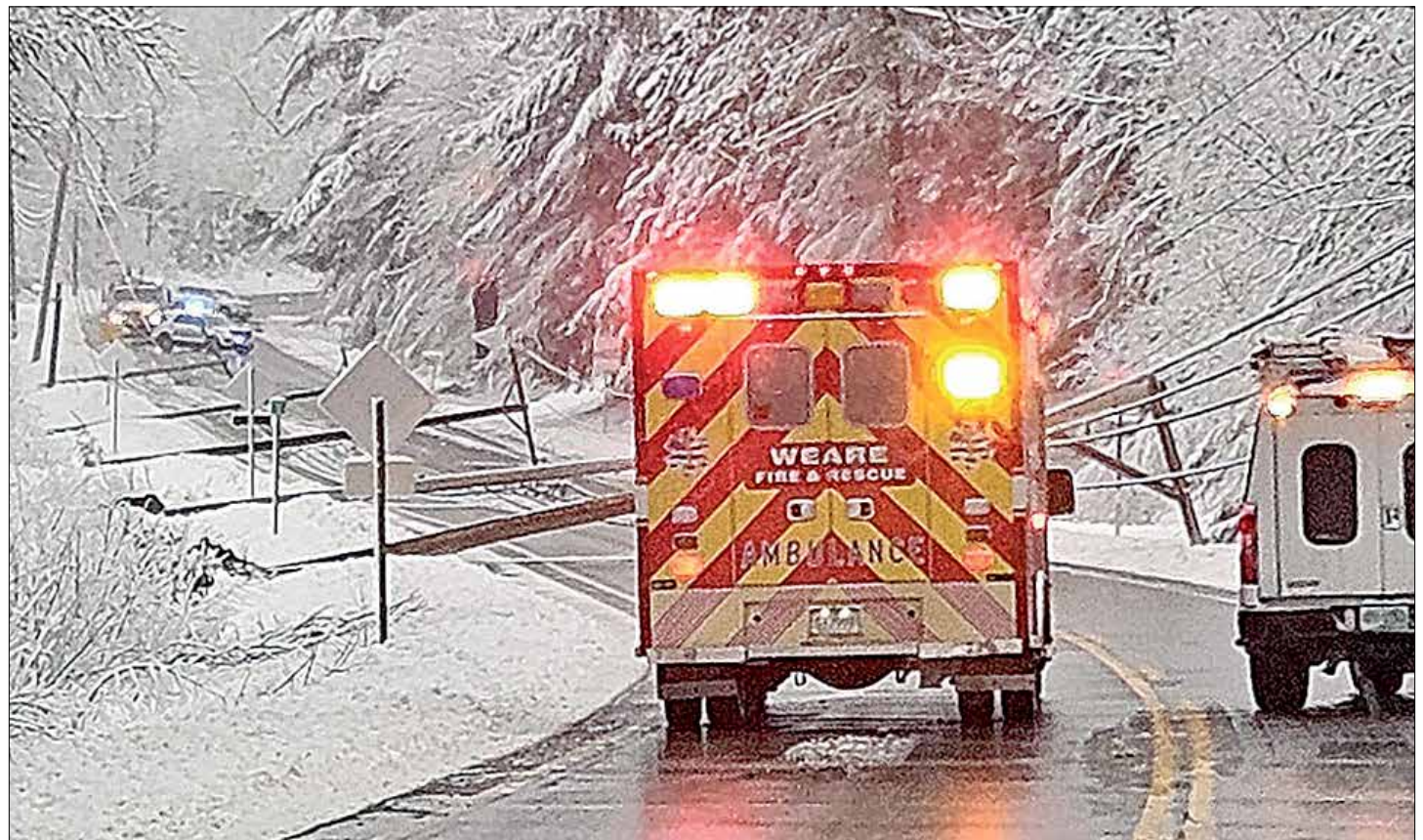
Multiple poles ripped from the ground on Route 114 in Weare shut down the road for an extended period during the last storm.
