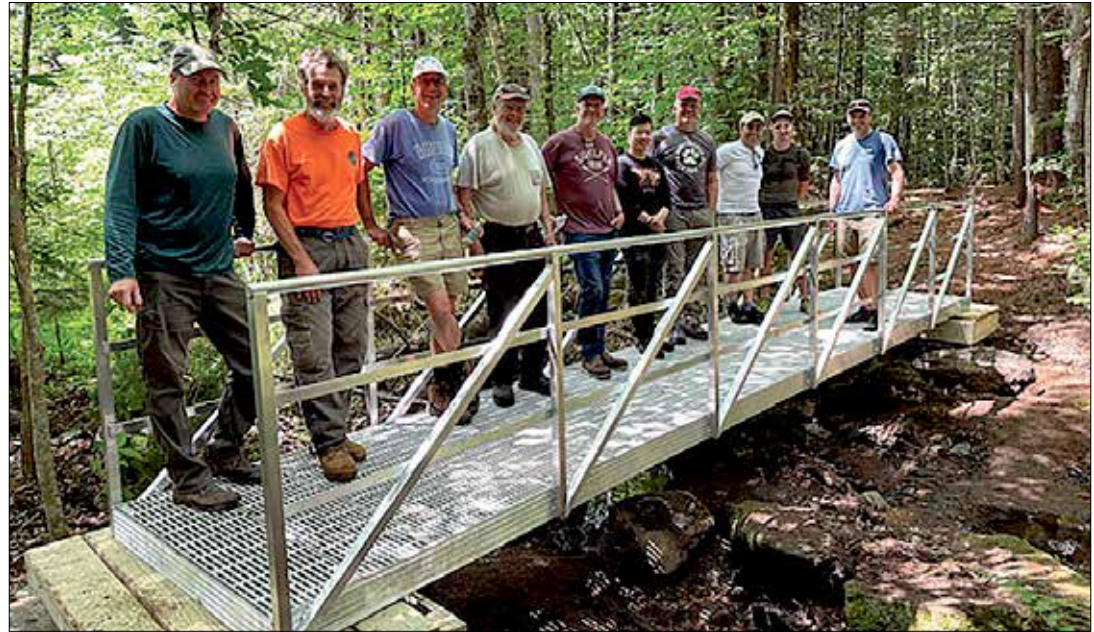
"On Friday the 26th, the New London Conservation Commission volunteers worked with a community service team from Hypertherm to install a 24-foot aluminum bridge on the Lyon Brook Trail. The new bridge replaces a decrepit wooden structure and completes a significant rehabilitation of the Lyon Brook Trail from Parkside Road to South Pleasant Street. The Commission thanks all of our volunteers and community partners for a job well done. We invite you to enjoy our trails!"
