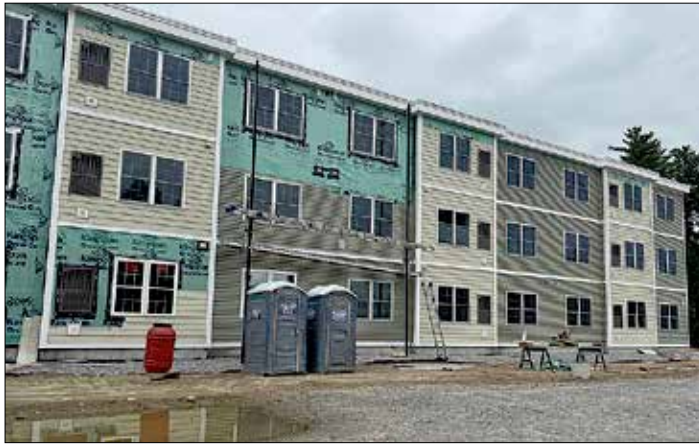
Avanru Development's Hillsborough Workforce Housing project is nearly 70% complete.
