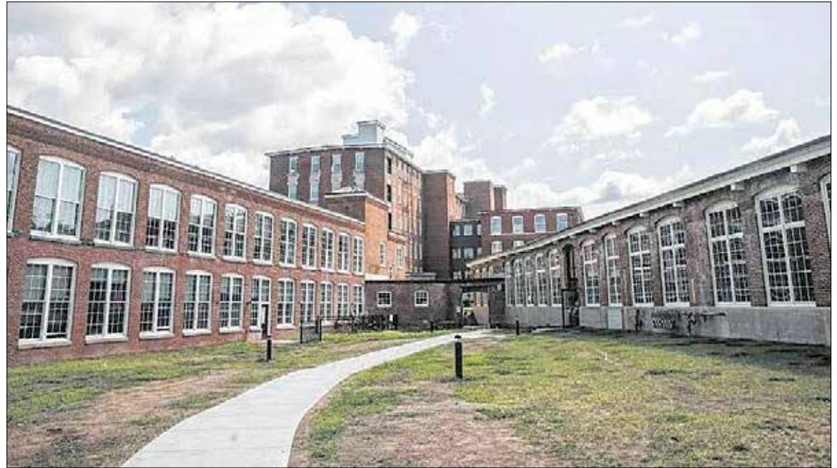
The renovated and restored Stevens Mills.
